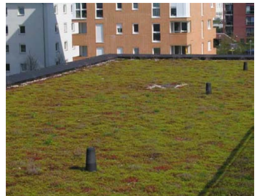
Grønt tak (Scharnhauser Park, Stuttgart).
