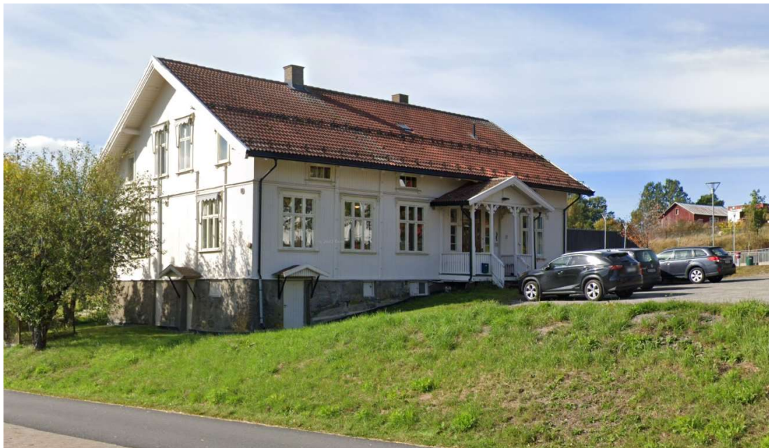
Figur 15 Hammer skole, eldre skolebygning. Kilde: Google Maps street view, september 2022.
