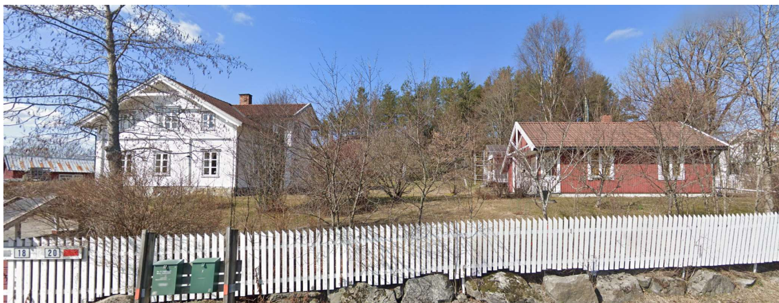
Figur 13 Søndre Hammer gård. Kilde: Google Maps street view, september 2022.
